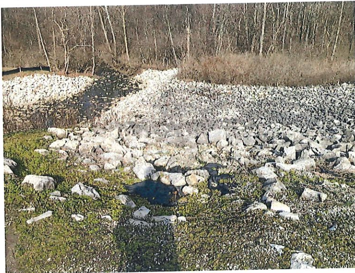
5. Portion of the right downstream slope covered with rock riprap.
