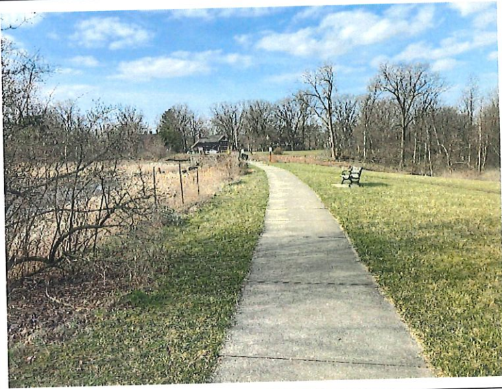
1. Overview from the right end of dam.
