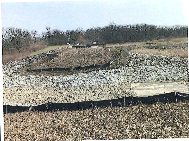
17. Overview of the emergency spillway channel.
