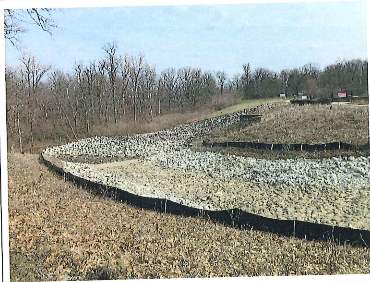
18. Overview of the emergency spillway channel.
