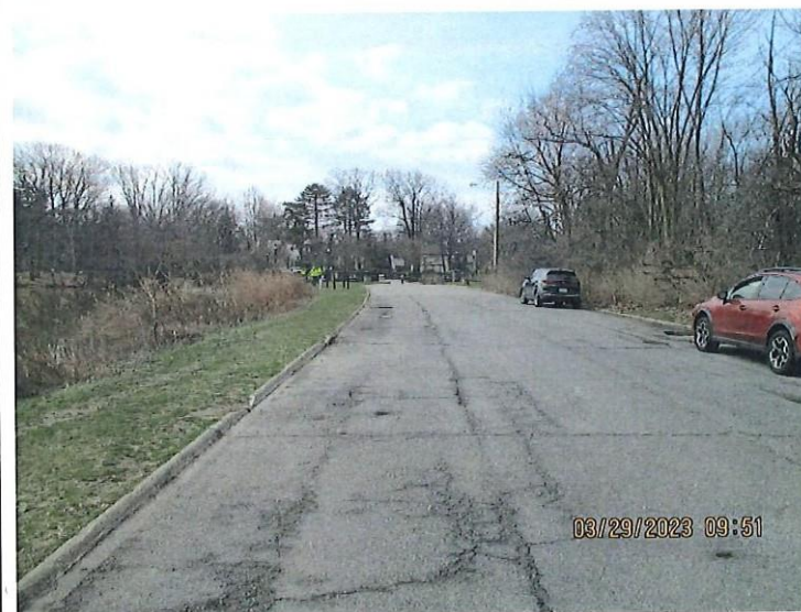
15. Overview of the crest looking toward the spillway.
