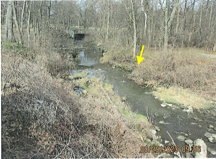
7. Channel downstream of the spillway; arrow points to the lake drain outlet.
