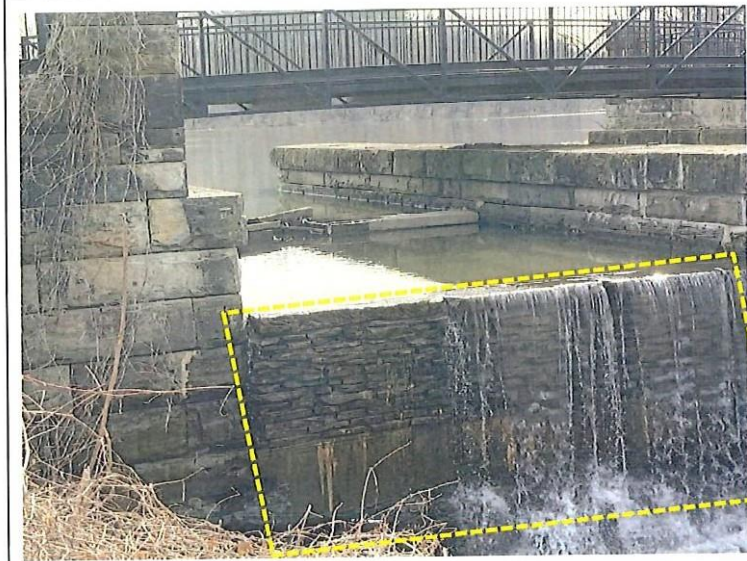
5. The downstream wall on the right side had recently been repaired.
