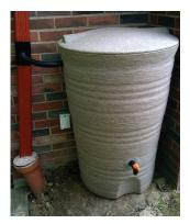
Example of rain barrel with downspout diverter that directs overflow back to the downspout
