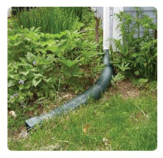
Examples of downspouts for vegetated filter strips
