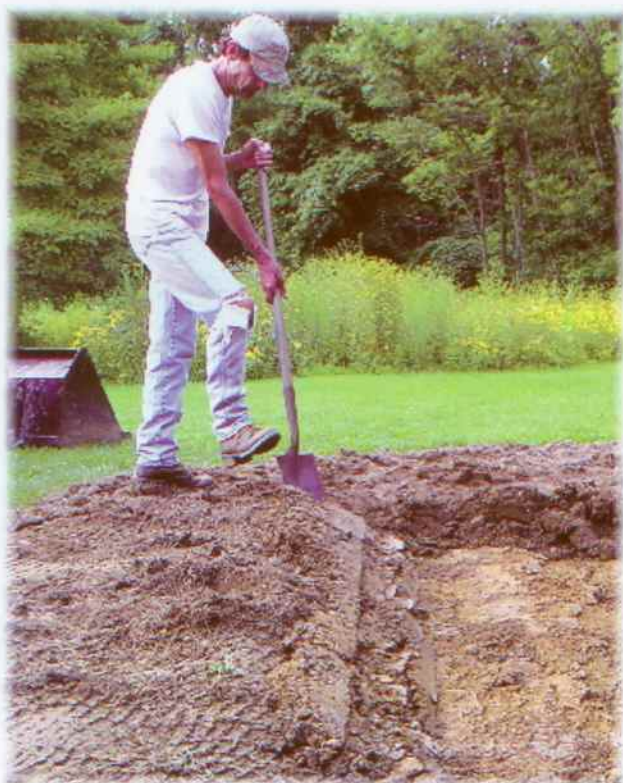
You can dig your rain garden by hand or use a backhoe. If you use a backhoe to dig your garden, avoid driving it on the garden site to minimize soil compaction.
