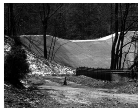
Figure 7-3 The flood detention basin on Doan Brook just downstream from Martin Luther King, Jr., Boulevard. Photograph by L.C. Gooch.
