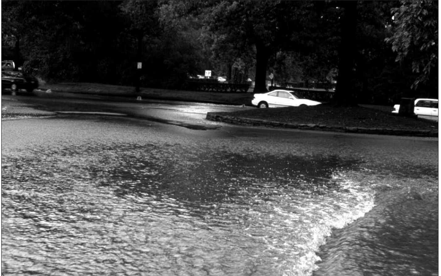
The Lower Shaker Lake dam overflows into North Park Boulevard. August 31, 2001. Photograph by L.C. Gooch.
