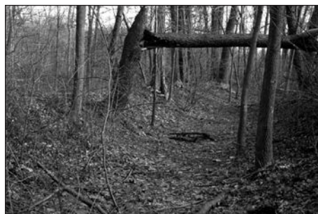
Figure C-3 Remains of the earth channel that once carried a wooden flume along the south side of Doan Brook between Horseshoe Lake and the Shaker woolen mill near South Park Boulevard and Lee Road. Photograph by L. C. Gooch.
